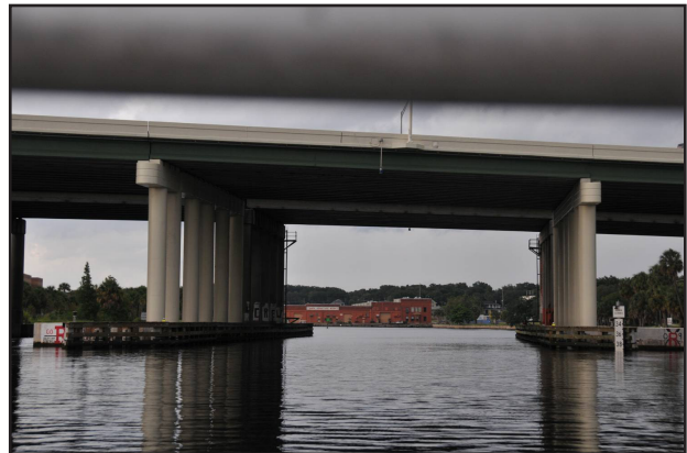
Figure 5: Looking northward through an overpass onto the site. Photograph by Shannon Bassett used by permission.
